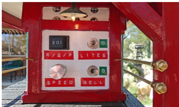
Conveniently labeled control panel behind Gear Room.
