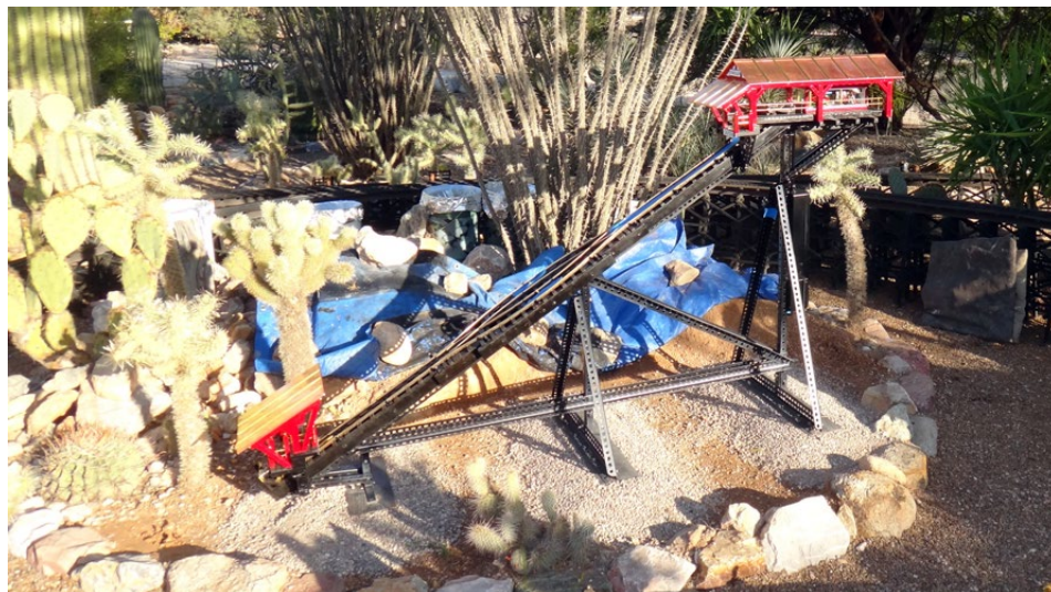
Funicular railroad tubular and angle iron structure set into footings before mountain building.
