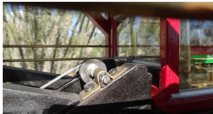
Two 7/8" stainless steel pulleys redirect their cables horizontally into a hole in the Gear Room's glass wall.
