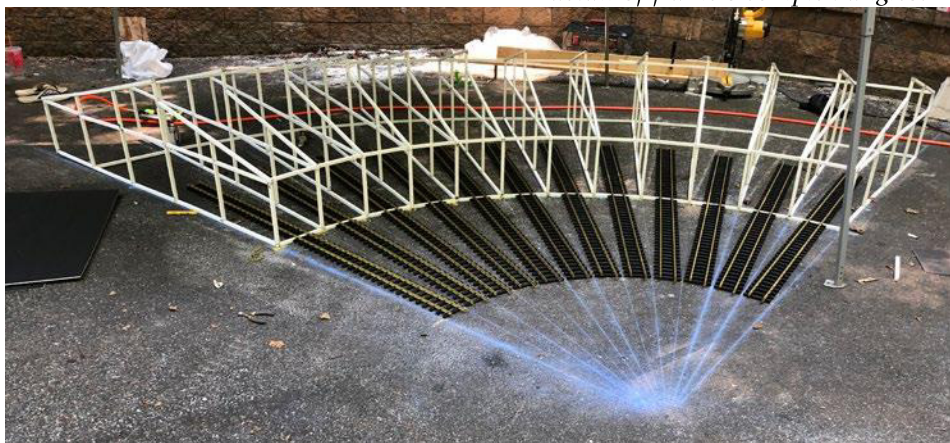
The framework of the assembled roundhouse. Track is placed for position.
