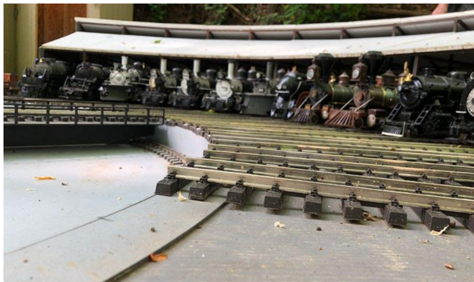
The first 12 bays of the Maryland Central RR roundhouse with walls completed and roof sheathing in place. Still to come are doors and roofing.
