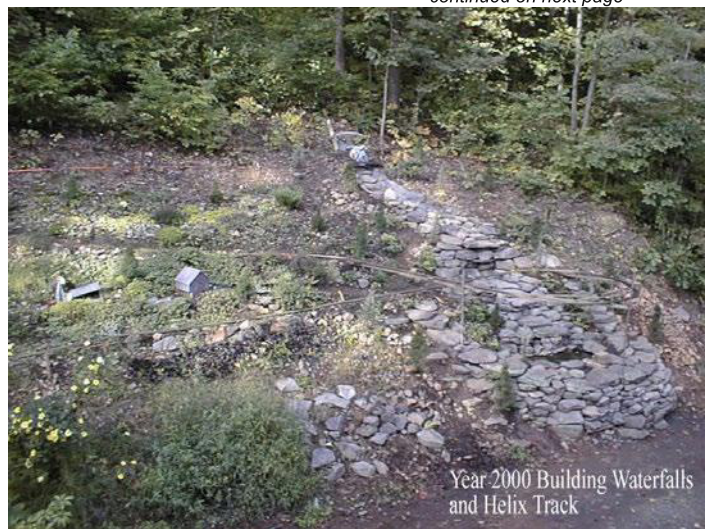
Construction of the waterfall included laying a helix loop over the pond and a loop along the top of the hill.
