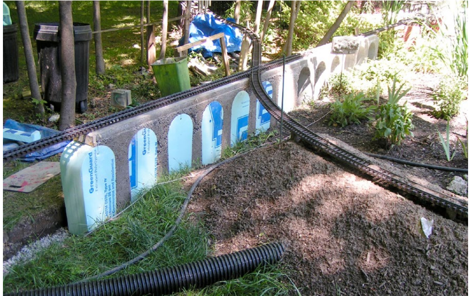
Fig. 8: First two sections poured
