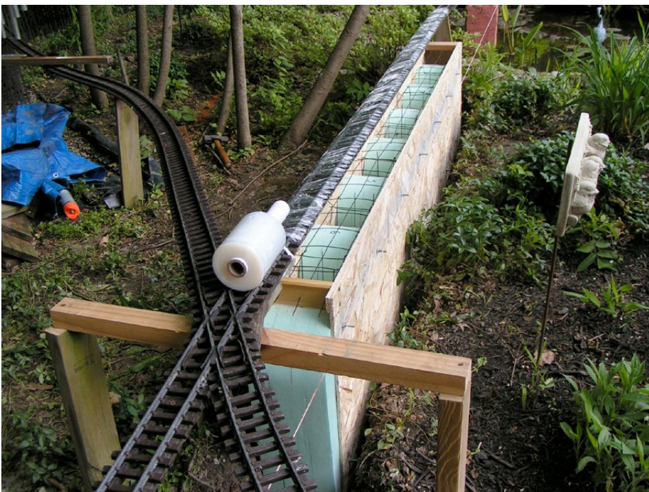
Fig. 5: First form, ready to pour. Note wire fence rebar between arches.
