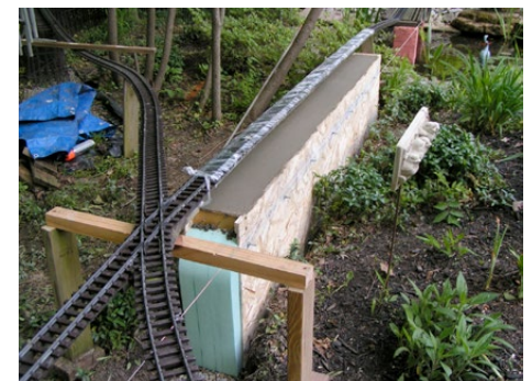
Fig. 6: The first section, poured
