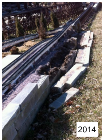
Frost Heave Damage
