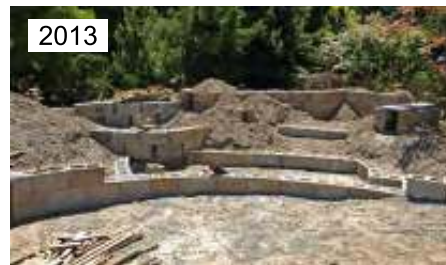
Layout #3: Pond and waterfall under construction.
