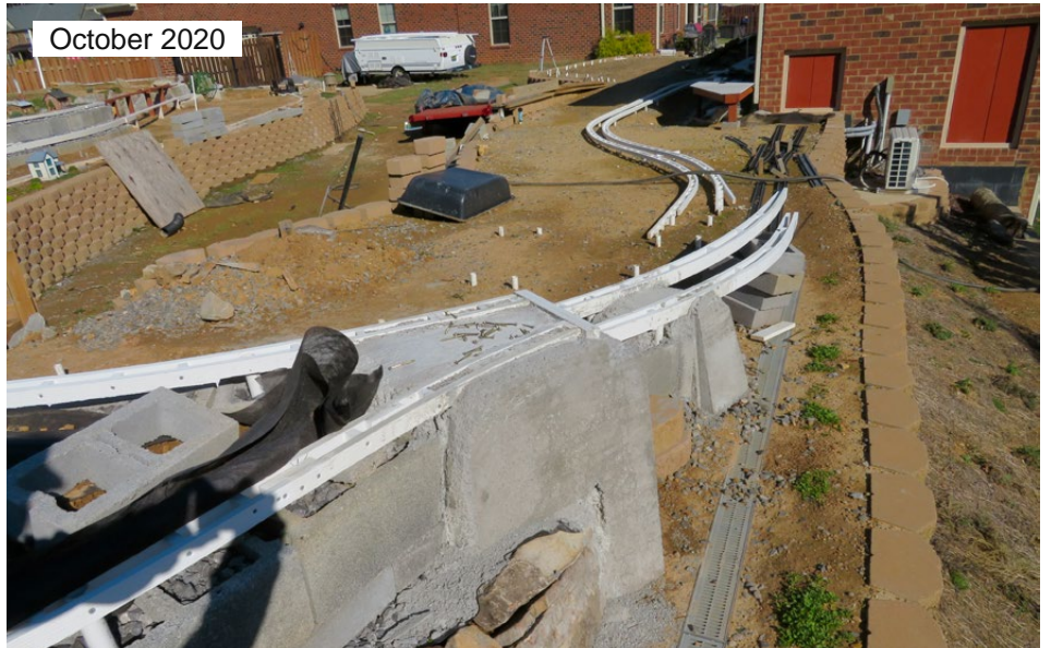
Below: Drainage grates along the retaining wall take rain to a pipe.
