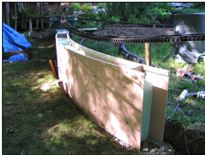
Fig. 1: Curved Form in Place
