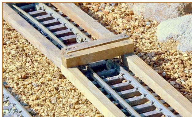
The ballasting frame for straight track; there was an articulated version for curved track.
