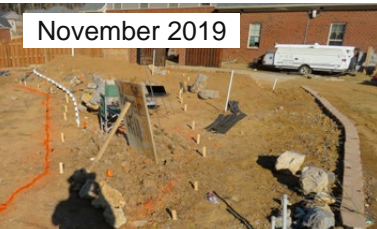
Grant set track stakes for ladder-style track bed in late 2019. Retaining walls and fill for hills went in that winter. Leveling track bed came next.
