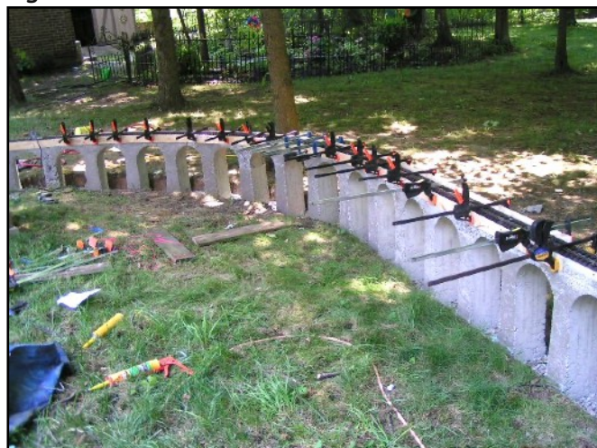
Fig. 2: OSB for Wall Material - FAIL
