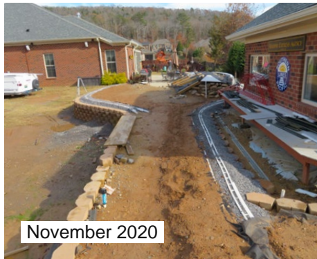
Above: Roadbed installation on the south lobe. Platform along the train shed will support upper level track.
