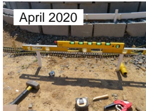
Grant set track stakes for ladder-style track bed in late 2019. Retaining walls and fill for hills went in that winter. Leveling track bed came next.
