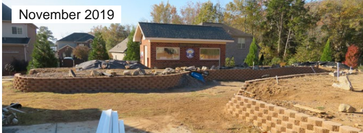
Grant set track stakes for ladder-style track bed in late 2019. Retaining walls and fill for hills went in that winter. Leveling track bed came next.
