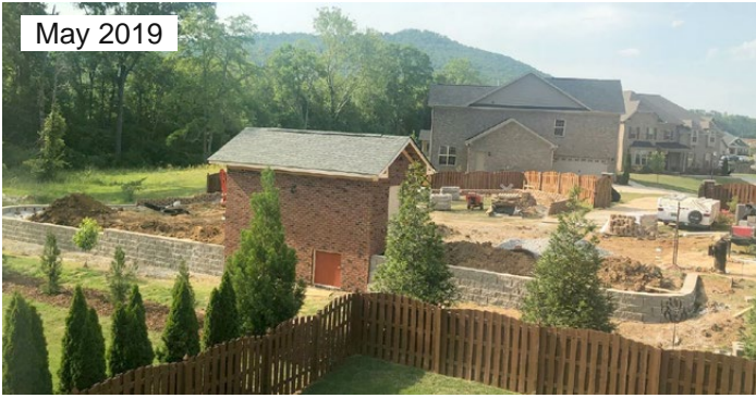
With the 3.5 foot retaining wall with drains in place, fill dirt started coming.
