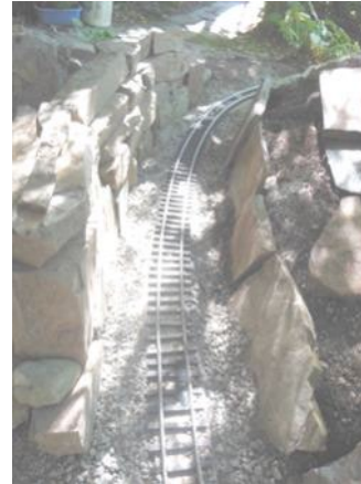
Track Prior to Roofing the Tunnel.
