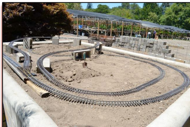
Track in place on temporary supports
