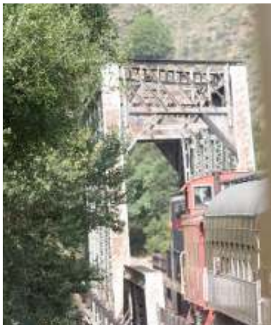
This bridge on the Niles Canyon Railway dates from 1908.
