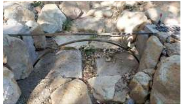
Photo 3 Test-fitting the first arch.
