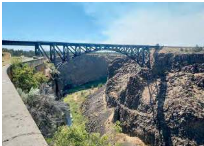
Photo 1 Crooked River Railroad Bridge.
