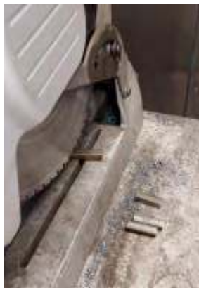
Photo 6 Cutting some of the shorter cross braces.
