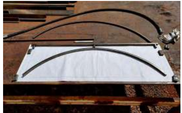
Photo 4 Checking the beginnings of one side against the drawing of the gap to be spanned.
