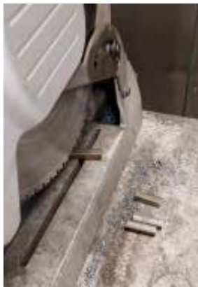
Photo 6 Cutting some of the shorter cross braces.
