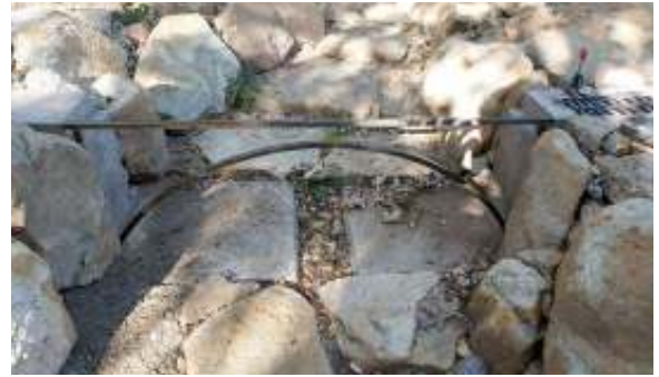
Photo 3 Test-fitting the first arch.
