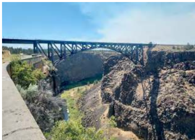
Photo 1 Crooked River Railroad Bridge.
