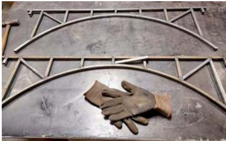
Photo 7 Fitting the cross braces.
