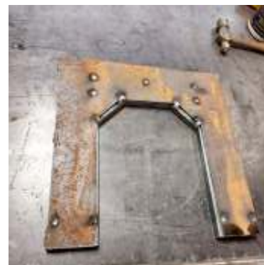
Photo 8 Welding the backing plate on.
