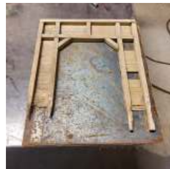
Photo 2 Transferring measurements onto the steel plate.
