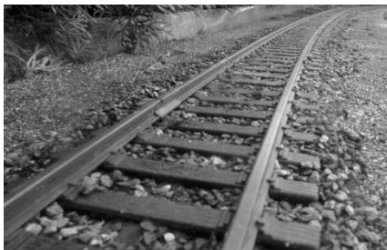
Track laid in 1997, still in perfect condition
