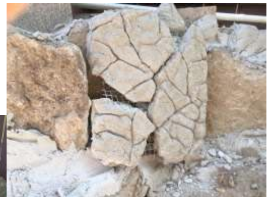
Tile ready to mortar in place ↘
