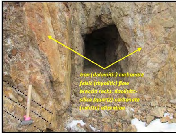
Photo 3: Old adit @ elev. 666 – part of Alice copper zone. Copper-bearing iron carbonate appears to be associated with altered felsic – rhyolitic unit. Dimensions of adit: 6m long x 1.25m wide (at the face) x 2.4m high. Black, broken lines bottom left trace altered volcanic-carbonate (dolomitic) strata, which strike and dip are similar to strata shown in photo 2.
