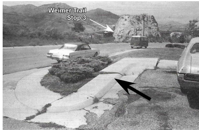
Fig. 102. Cracked and slumped sidewalk (black arrow) on the CSM campus circa 1977, caused by differential subsidence. Today's Stop 3 on the Weimer Geology Trail (white arrow) in background. Photo from Amuedo et al. (1978, p. VI-6a). View to north.
