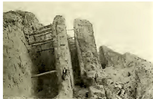
Fig. 78. Log “strain gauges” at the Hoyt Mine in 1901 with a man for scale. Photo from Geijsbeek (1901, p. 243).
