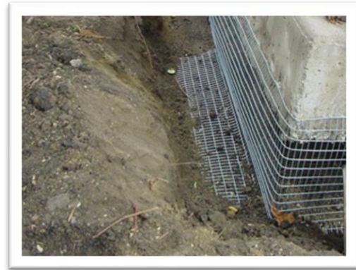
L-shaped screen prevents predator digging
