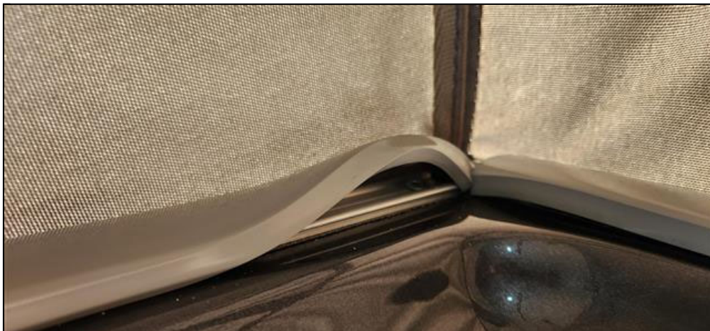
Trim In Bunk Area
