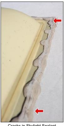
Cracks in Skylight Sealant
