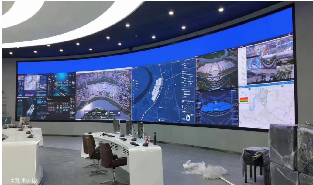
P1.25 LED display for central control room
