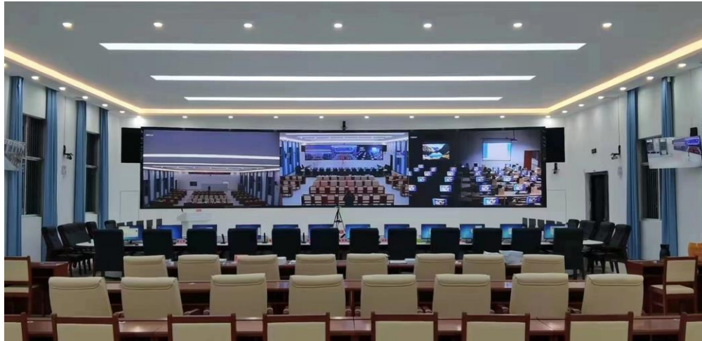
P1.538 LED display for central control room
