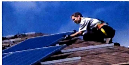
Solar Panel Installation
