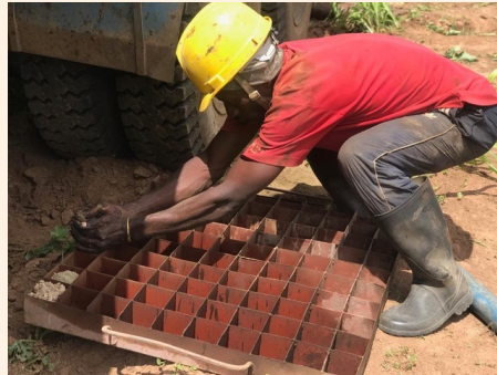
Ndebwe villager laying the foundation
