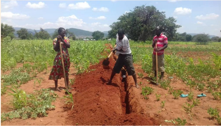
So far 800 meters of trench has been dug.
