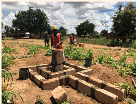
Laying foundation for the tower
