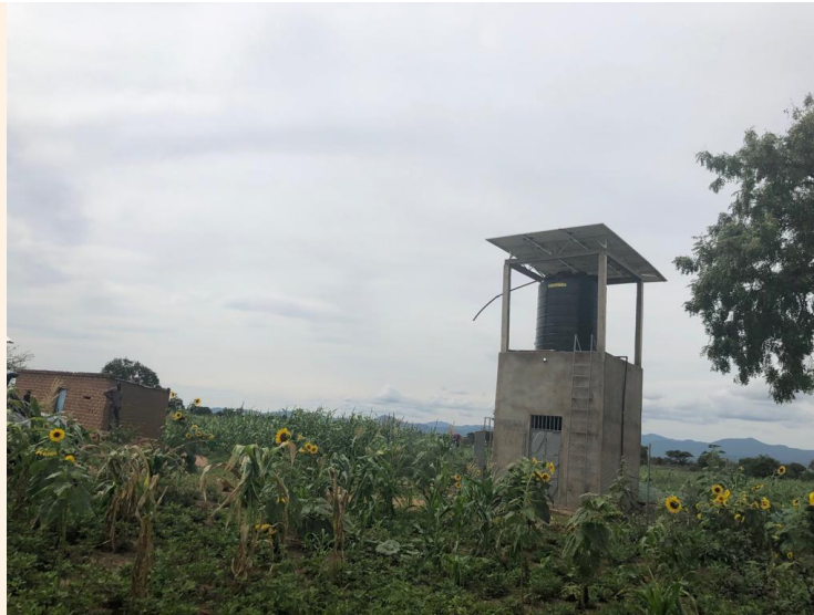
Solar Technology Pumps 20,000 Gallons of Clean Water Daily for Mwinyi Village
