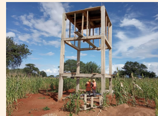
Ndebwe Villagers building the Water Tower
