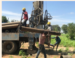
Laying the Piping
