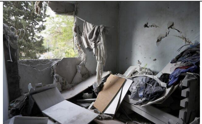
A picture taken early on May 11, 2021 shows a damaged building in the southern Israeli city of Ashkelon after rockets were fired by the Hamas terror group from the Gaza Strip towards Israel overnight amid spiraling violence (JACK GUEZ / AFP)
