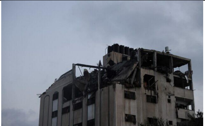
Parts of an apartment building is destroyed following Israeli airstrikes in the Gaza Strip on May 11, 2021 (MOHAMMED ABED / AFP)
