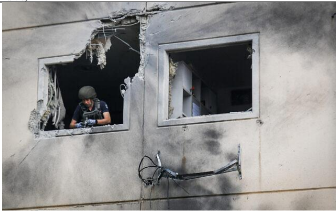
An apartment building that was hit by a rocket fired from the Gaza Strip in the city of Ashkelon on May 11, 2021. (Flash90)
