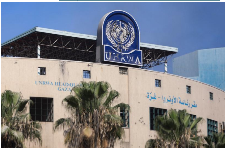
A damaged sign is pictured at the headquarters of UNRWA, following an Israeli raid, amid the Israel-Hamas conflict, in Gaza City, July 12, 2024. (credit: REUTERS/DAWOUD ABU ALKAS)
