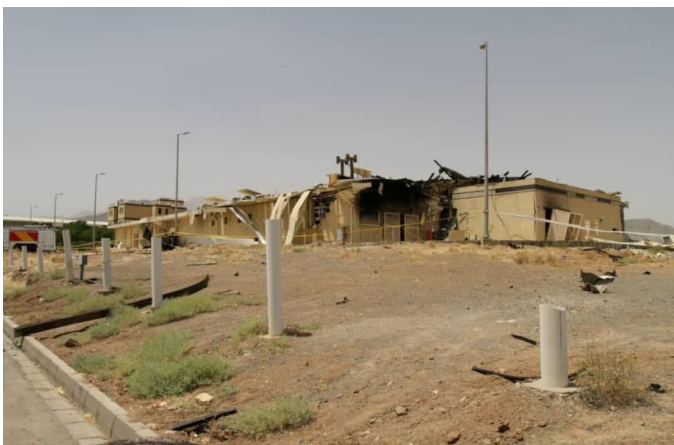
VIEW OF a damaged building after a fire broke out at Iran's Natanz Nuclear Facility, in Isfahan on July 2.(photo credit: ATOMIC ENERGY ORGANIZATION OF IRAN/WANA VIA REUTERS)
