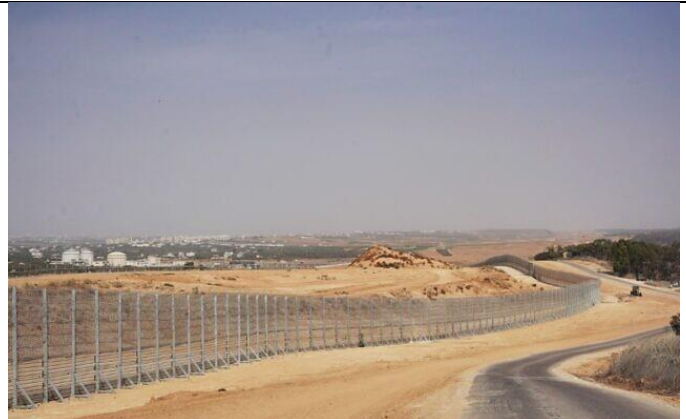
A portion of the 40-mile barrier along the Gaza Strip, upon completion on December 7, 2021. (Defense Ministry)
