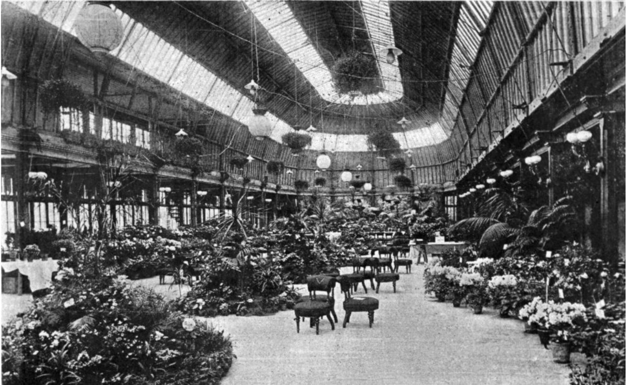
(Above: Notice the new chaotic electrical wiring hanging from the ceiling.)
