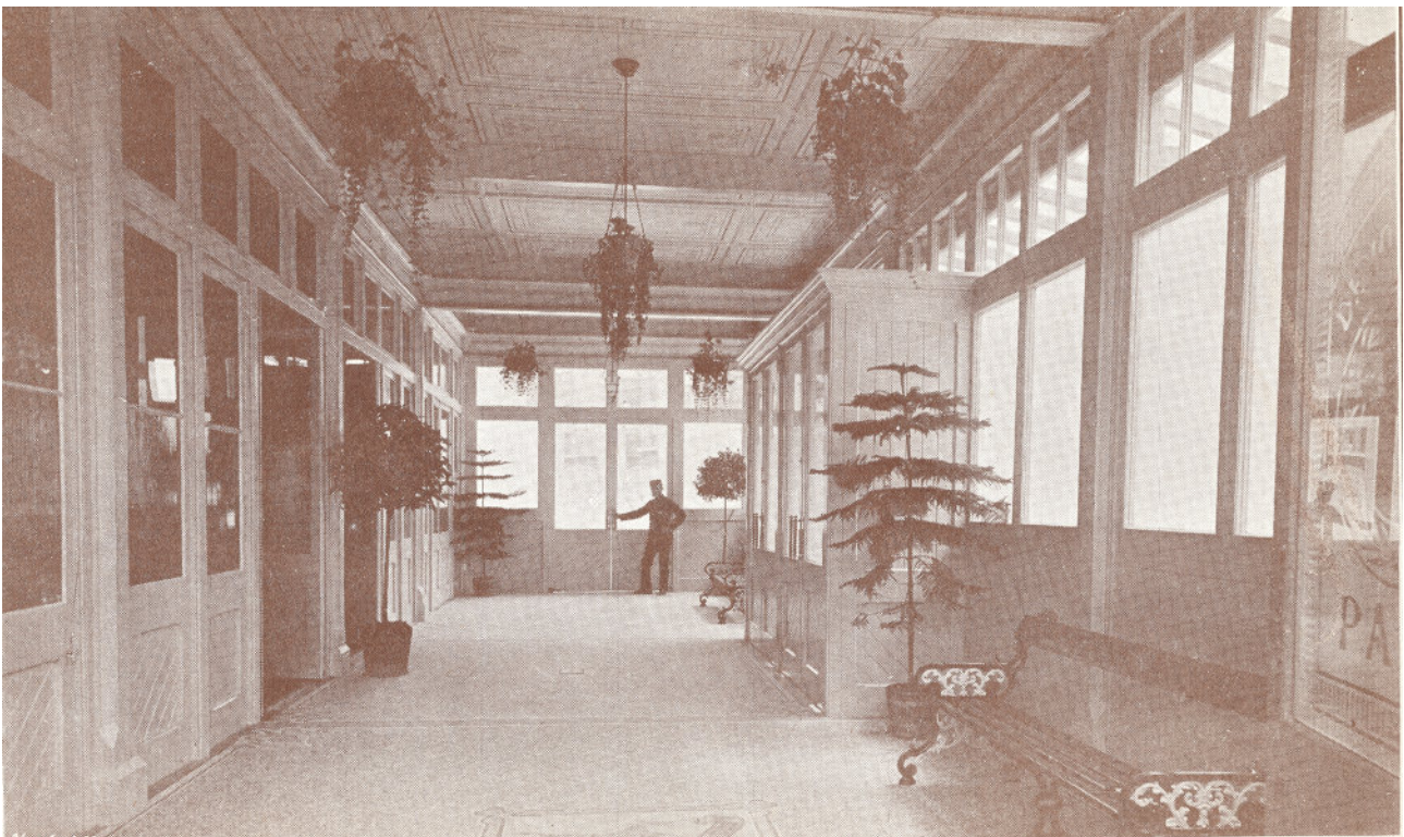
(Above : The new Portico. This was previously the covered carriageway.)
