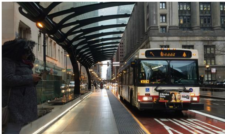
Figure 28: New Loop Link busway, downtown Chicago. Possible model for Fayette and Baltimore
