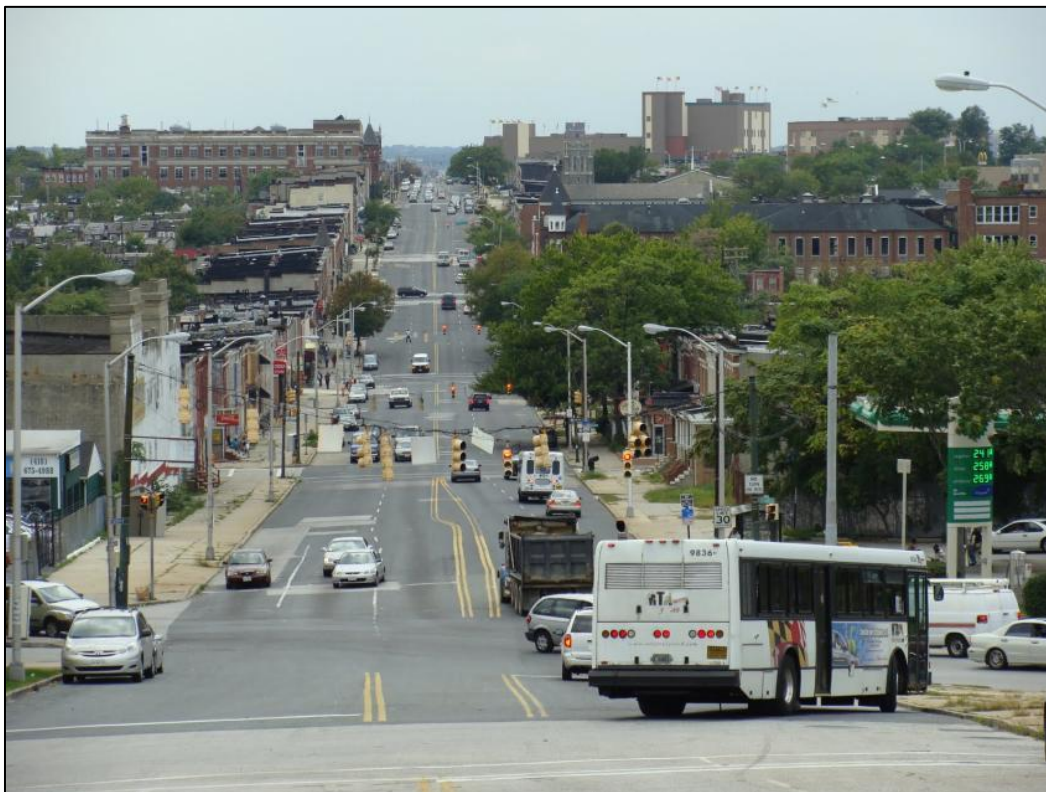
Figure 42: North Avenue has a classic pre-BRT configuration for much of its length, and width varies from block to block
