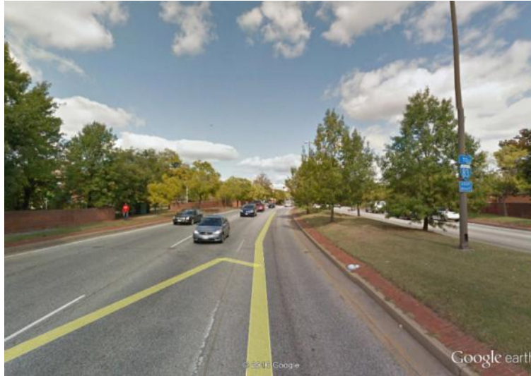
Figure 58: MLK Blvd between Route 40 and Eutaw Pl has a median and additional ROW that could accommodate BRT.
