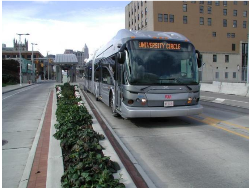
Figure 24: Dedicated bus lane in the middle of an urban arterial, Cleveland HealthLine BRT
