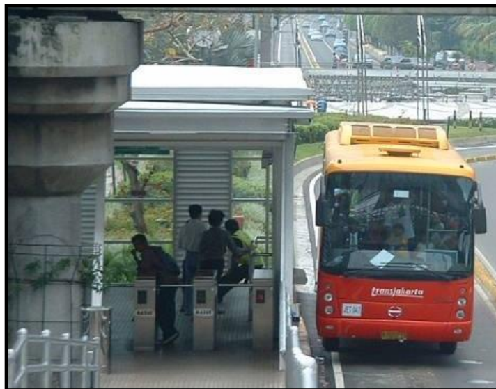
Figure 32: Gate controlled BRT Station, Jakarta, Indonesia
