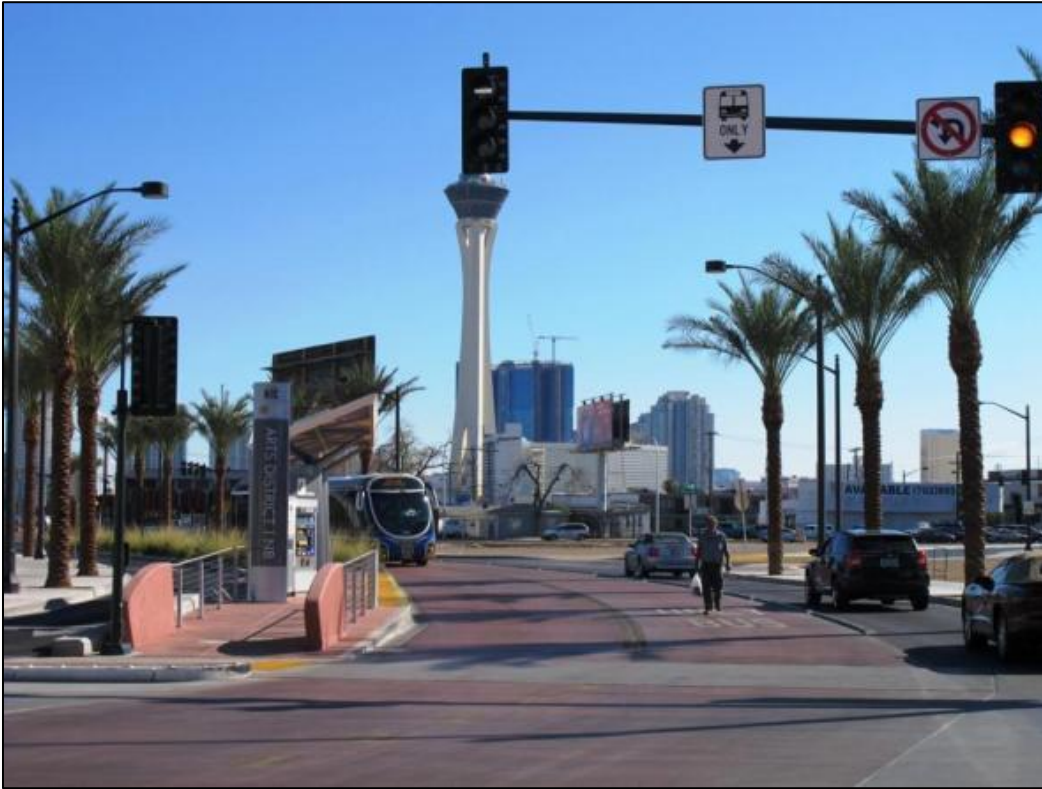
Figure 34. Median BRT on an urban arterial in Las Vegas. Most left turns across the busway have been banned.
