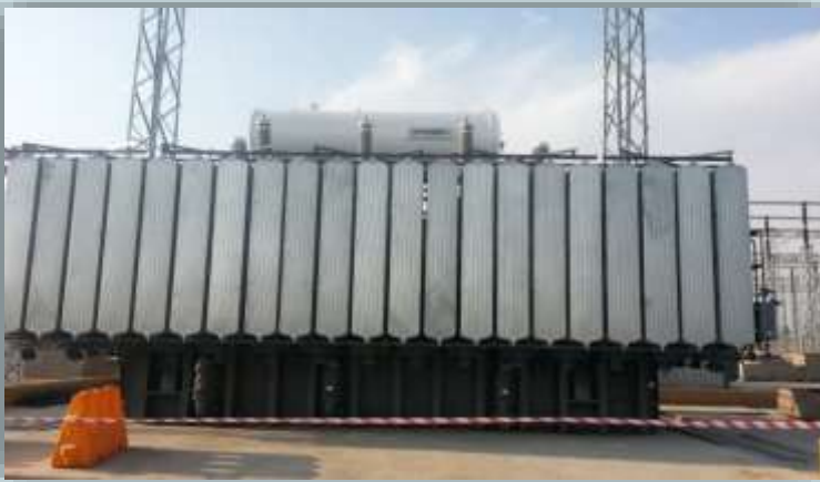
Borutho substation (Hyundai 500 MVA Trfr)
