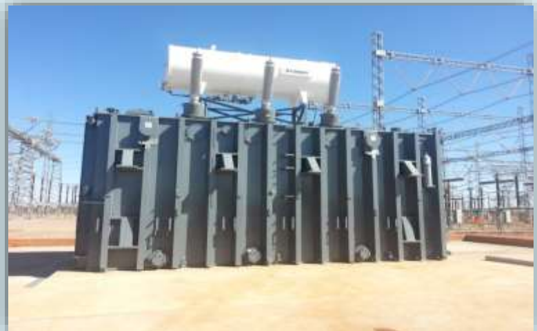
Spitskop Substation (Hyundai 500 MVA Trfr)
