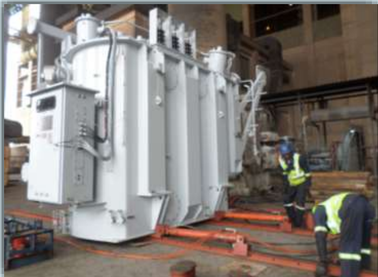
Duvha Power station (Hyundai 770 MVA Trfr)
