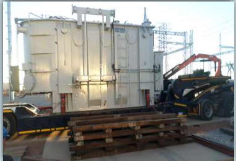
Matimba Power station (Powertech transformers 40 MVA
