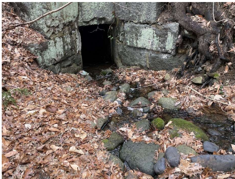
There are several existing stone block culverts along the corridor which facilitate storm water flow.
