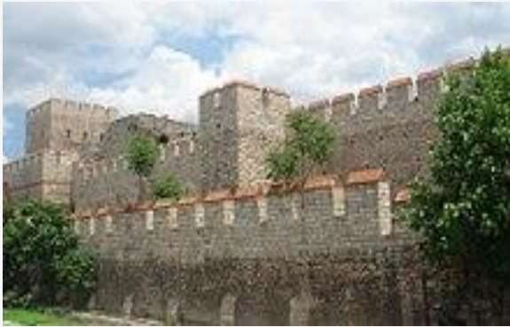
Walls of Constantinople
