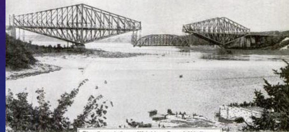
The Central Span, Weighing Over 5,000 Tons, being Raised by Practically the Same Method as was Employed Last Year, with Certain Added Precautions
