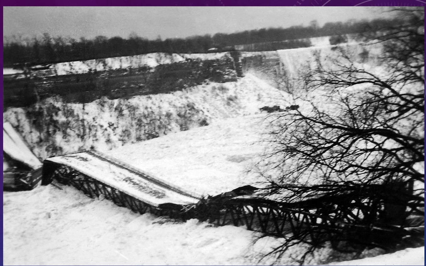
A sudden wind storm on Lake Erie sent a massive amount of ice over the falls, resulting in nearly 100 ft (30 m) of ice pushing against the bridge.
