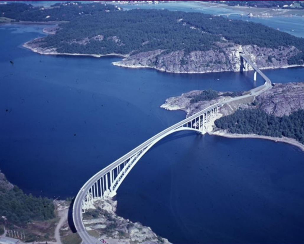
The Almö Bridge in 1962, Stenungsund, Sweden, 18 January 1980, Steel arch bridge
