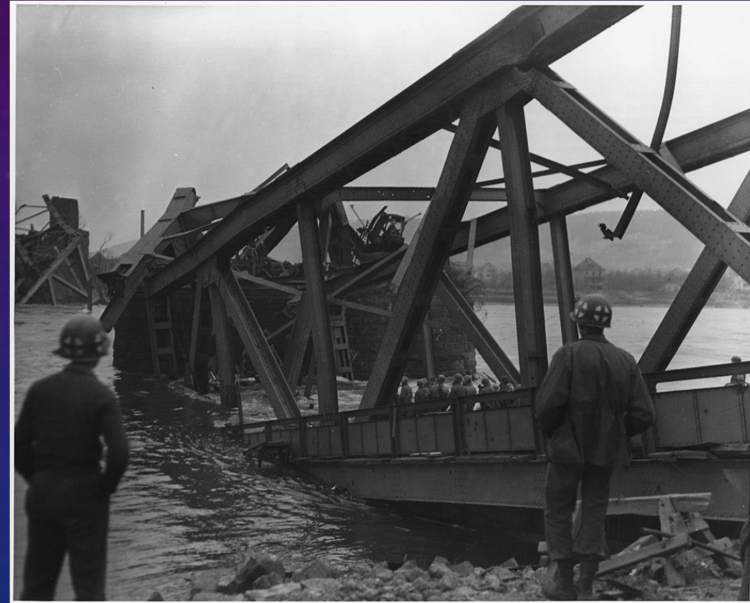
Ludendorff Bridge on March 17, 1945 after the collapse, Collapse due to previous battle damage incurred 7 March 1945
