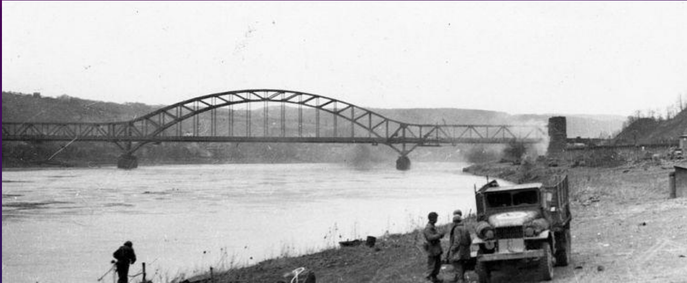
Ludendorff Bridge (Remagen Bridge) side view Germany
