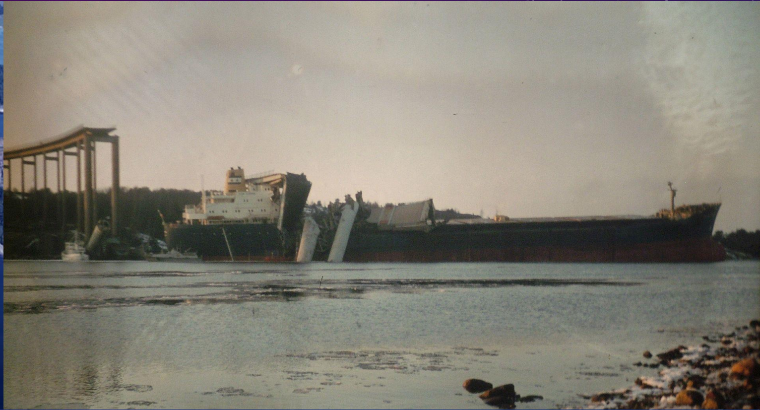
The collapsed bridge and MS Star Clipper Ship collision during bad visibility (mist)
