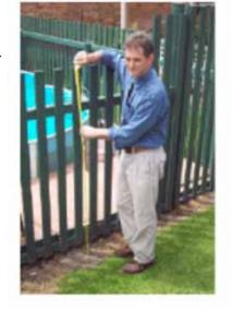
to prevent access, or the steps or ladder can be surrounded by a barrier, such as those described above. For any pool barrier, the maximum clearance at the bottom of the barrier should not exceed 4 inches above grade, when the measurement is done on the side of the barrier facing away from the pool.
