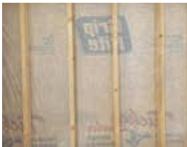
Tyvek House Wrap in Walls
