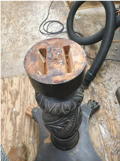
The second set of photos are of a second Empire table base which I “inherited” without a top. The block on which a top would sit was doweled on with four 1/2” dowels and did very little to hold the block in place. Traditional construction is a double tenon and that is what I recreated with this “new” splice.
