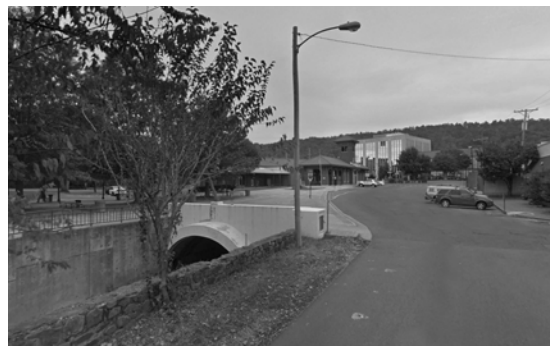
Existing culvert and stream channel on Broadway Terrace
