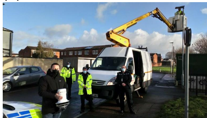
(Police Community Support Officer (PCSO) Tom Palfrey, PCSO Carlos Paulo, Inspector Ruth Atherton and Dan Stokes from Wireless CCTV Ltd with one of the new CCTV cameras installed)
