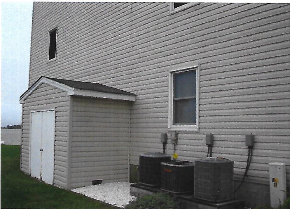
Left Side View of #120 53 rd Street (Building #1 – see attached plan) on 9-30-2016.
