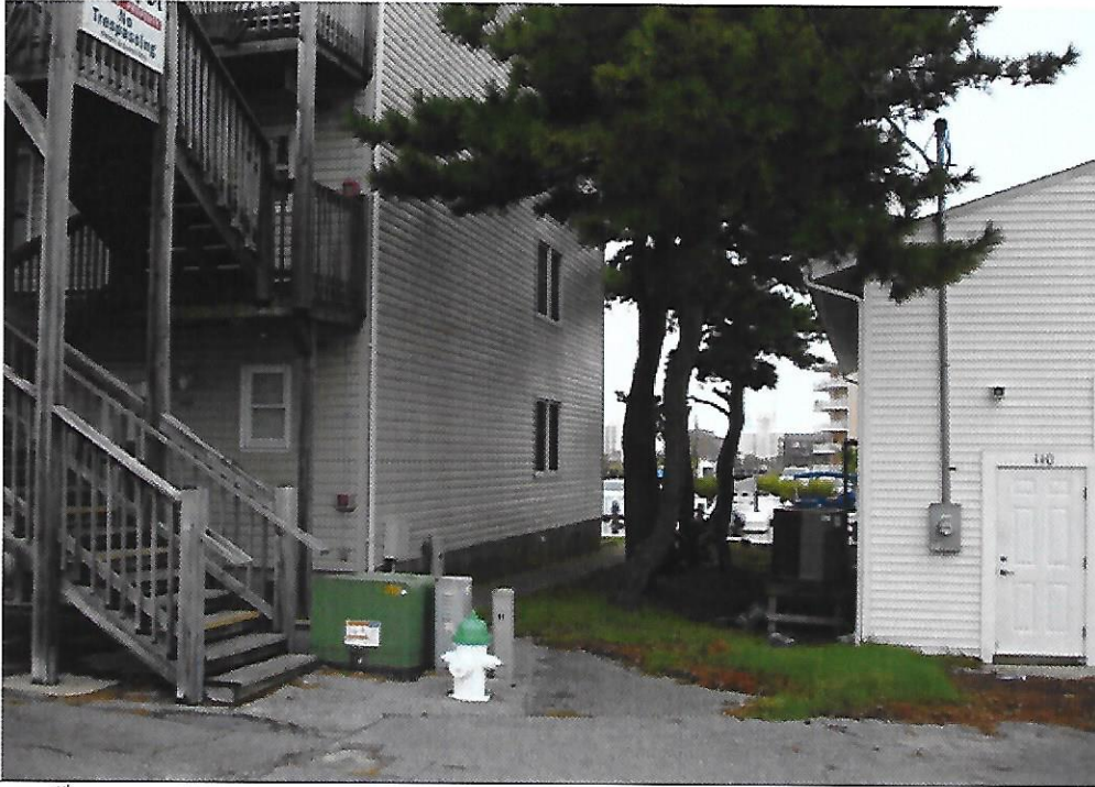
Right Side View of #120 53 rd Street (Building #1 – see attached plan) on 9-30-2016.
