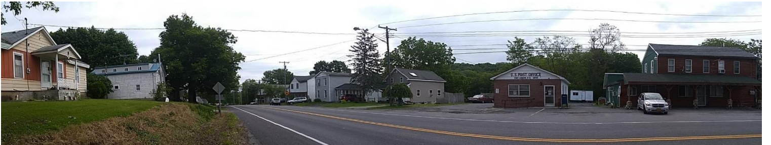
Figure 9g. View NE to E on Atwater, N of Grieg. Historic commercial corridor. Note variegated cladding, often non-historic (e.g. faux-log at far R, brick and vinyl on post office); frequent altered fenestration and form, including added dormers, porches, etc.
