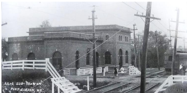
Figure 5. RS&E structure from SW, c. 1910; note trolley car at far R
