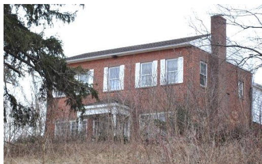
Figure 8. Field House (105 Field St.); note altered fenestration, loss of stepped gables and replacement w/ vinyl clad pitched gables
