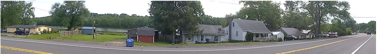
Figure 9a. View N to NE along Route 31 near W intersection w/ county line – mid-twentieth century canal-side cottages. Modern materials, dissimilar spacing, massing, and form throughout
