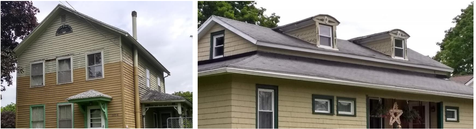
Figures 16a&b. Well-preserved architectural details that hint at hamlet’s history and help build sense of place along with density: fan ornament, hood brackets, and modest porch spindling and decorative brackets at 2958 Grieg St.; unique segmental arch dormers with decorative wood surrounds at 2948 Grieg St. While additions that obfuscate historic form and use of non-historic materials make these properties not eligible for National Register listing in our estimation, their adjacency compounds their surviving details’ contribution to the character of the hamlet.
