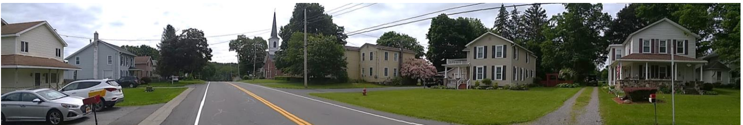
Figure 9d. View E to SE from Grieg St. W of Granger. Note altered fenestration (e.g. far L), modern materials (vinyl siding, added porches).
