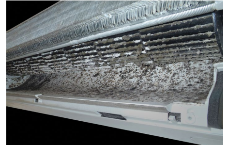
Mold thrives on mini-split blower wheels
