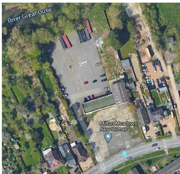
Figure 2 – Milton Meadow site from Google Earth showing development was on a site previously developed for commercial purposes.
