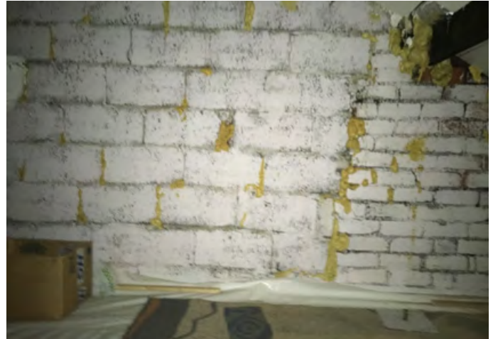
Figure 4 – expanding foam in all the cracks and in the top right of the image around the purlin.
