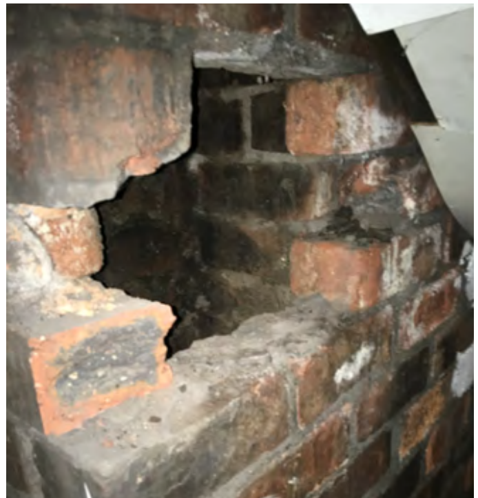
Figure 5 – hole in chimney (note the rough hole with no consideration for structural support of the chimney stack).
