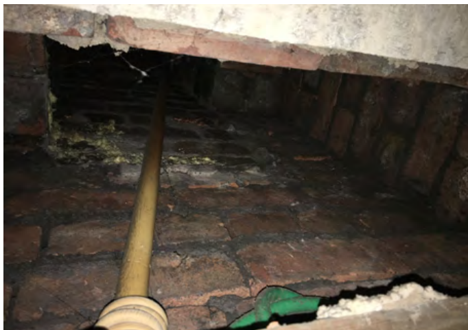
Figure 2 – bottom of chimney stack opened.
