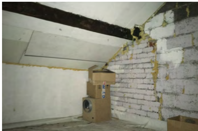
Figure 3 – plastic sheeting to the floor, roughly boarded over rafters and expanding foam to fill cracks.
