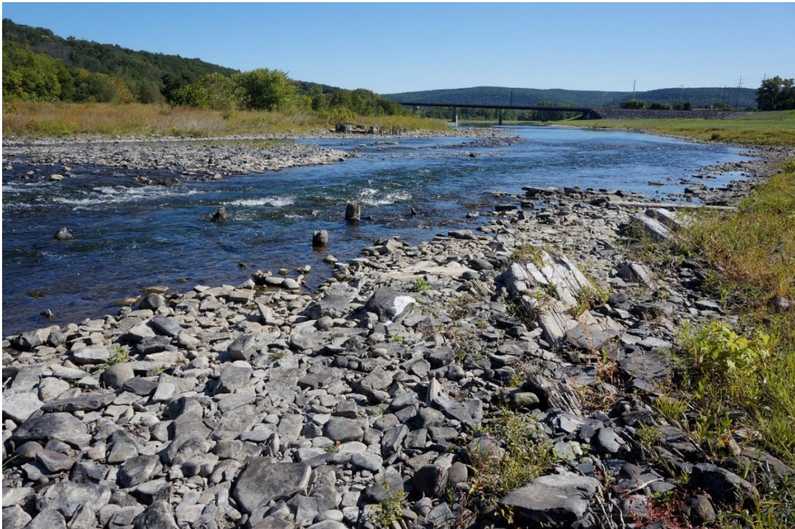
Figures 15 (top) and 16 (bottom). Top looking east towards Gibson over the line of piles that supported the feeder dam's foundation. Bottom showing dam timbers along west bank and in the center distance the pilings for the road bridge shown in Figure 13.
