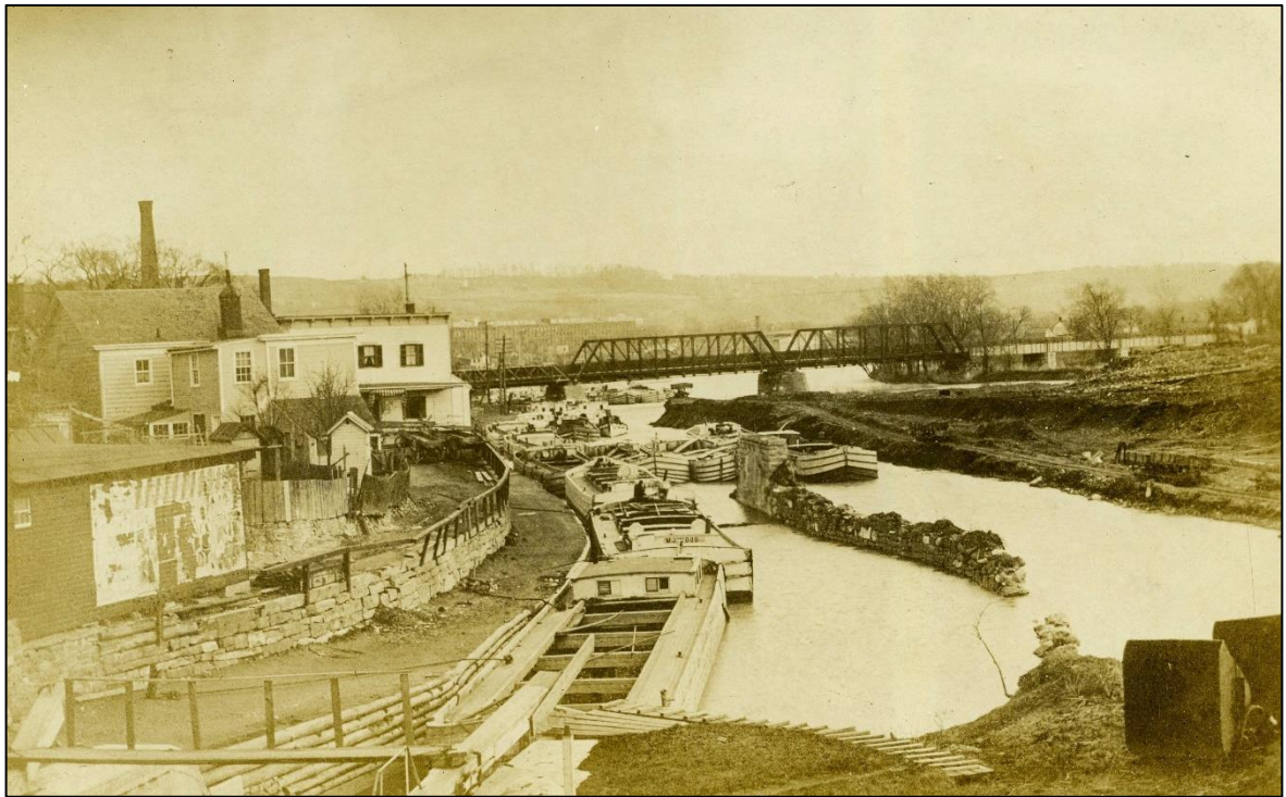
Figures 14 (top), 15 (bottom). Boats waiting below Waterford sidecut locks with construction of Erie Barge Canal Lock 2 underway, c1908.
