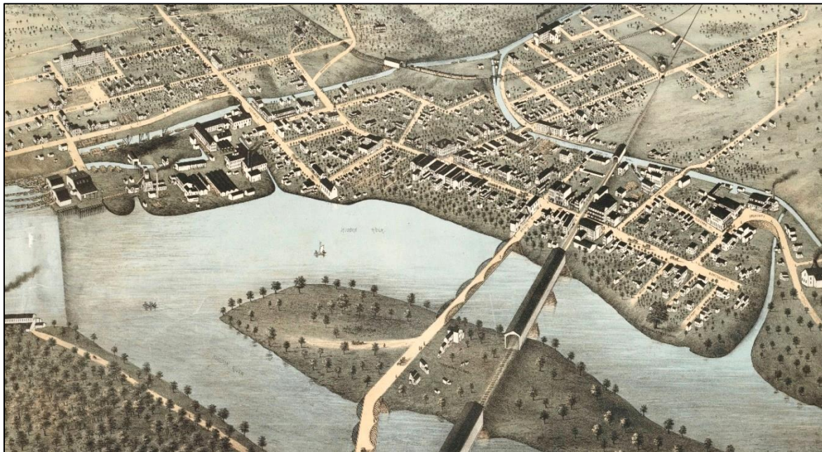
Figure 46 (top). Schillner map showing southern portion of Fort Edward, showing in darker shading the side canal to the Hudson River of the first Champlain Canal, 1896; Figure 47 (bottom). Detail of bird's-eye view of Fort Edward, 1875.
