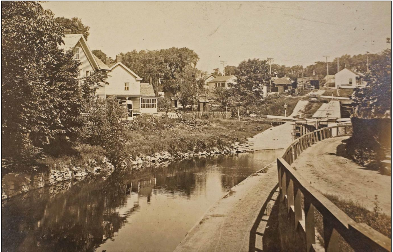
Figure 13. Looking west over the site of Erie Barge Canal Lock 2 with the Waterford sidecut locks to the right, c1905 (New York State Archives).
