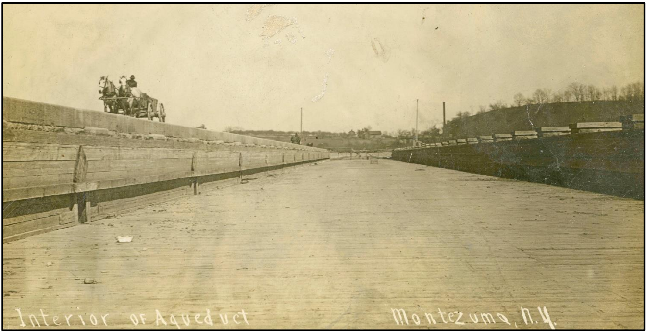
Figure 46 (top). Looking west along the north face of the Richmond Aqueduct, c1905; Figure 47 (bottom). Looking east through the dry trunk of the Richmond Aqueduct, c1917.
