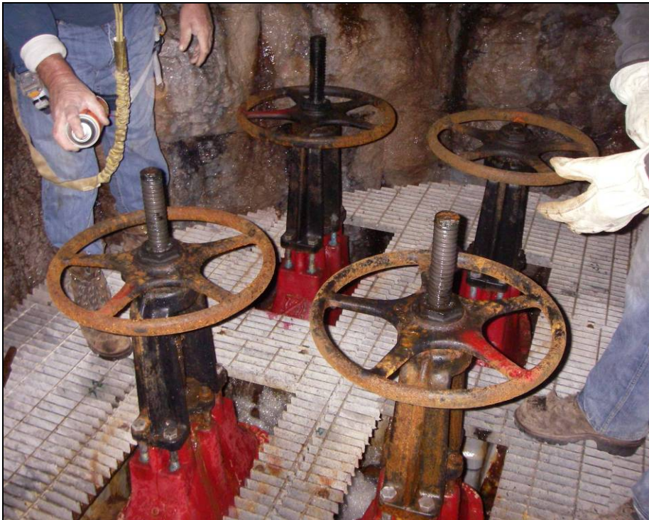
Figure 48 (top). Discharge valves of the DeRuyter Reservoir, 1862.
