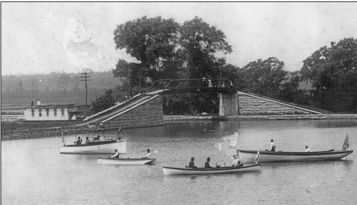
Figure 11 (top). Limestone Creek Aqueduct, looking south, c1910.
