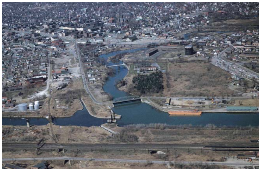
Figure 26. View from the south overlooking the junction of the Enlarged Erie and the Barge Canal, c1959 (CSNYS).
