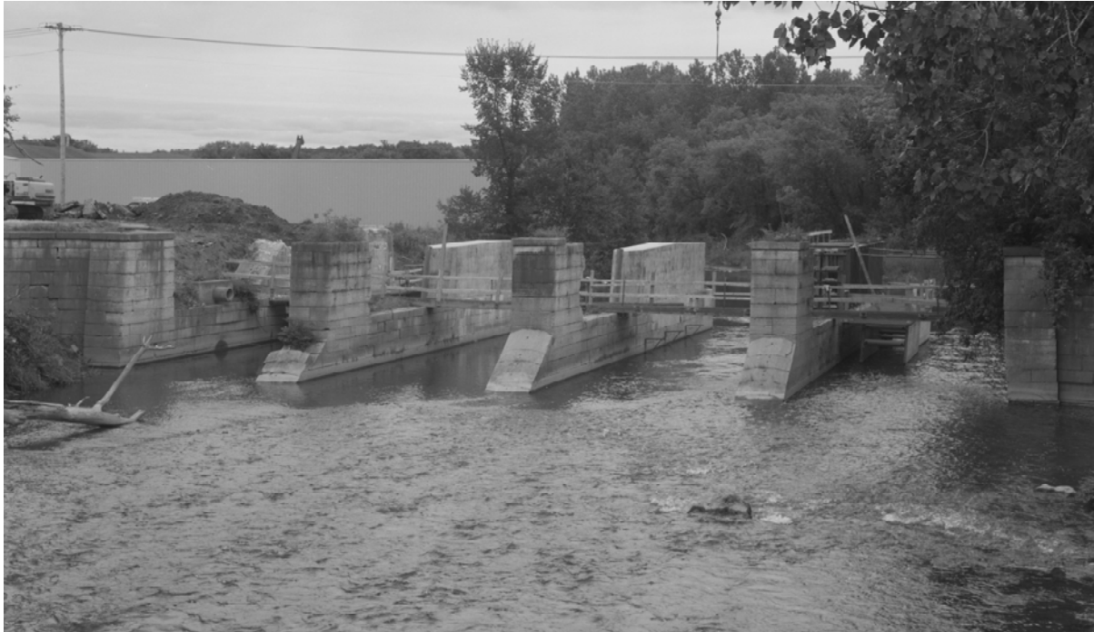
Figure 22. Enlarged Erie Oriskany Aqueduct during 2000 rehabilitation (CSNYS)
