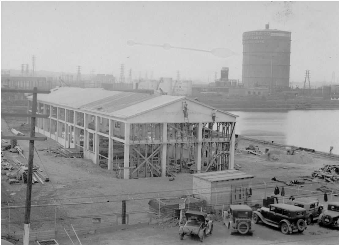
Figure 10. Constructing the Utica shop building, 1933 (New York State Museum).
