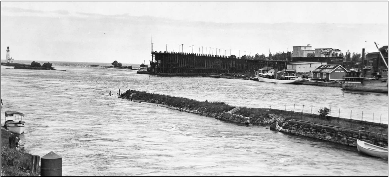
Figure 18 (top). Looking northwest over the prepared site for the State's Barge Canal Terminal at Oswego, March 18, 1918; Figure 19 (bottom). Looking northeast at Barge Canal Terminal at Oswego with the 1919 Barge Canal freight house to the right, June 15, 1922.
