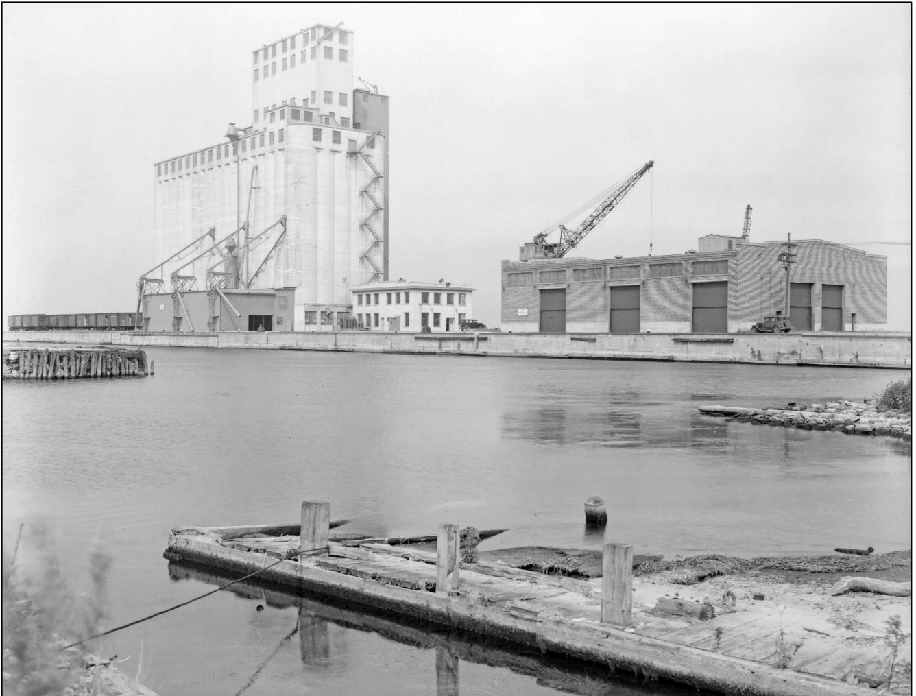
Figure 13 (top left). Grain elevator administration building under construction, August 21, 1924; Figure 14 (top right). Grain elevator administration building, May 18, 1925; Figure 15 (bottom). New York State Barge Canal Grain Elevator complex, looking northeast, c1930.
