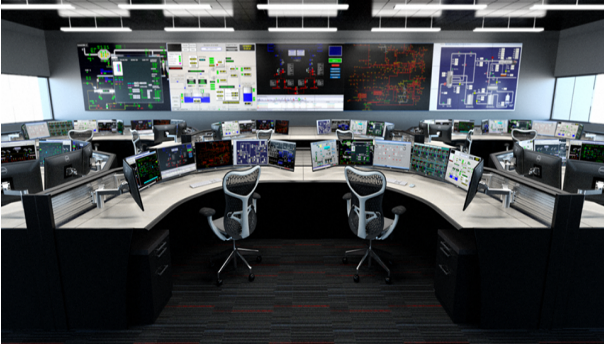
Command and Control Rooms
