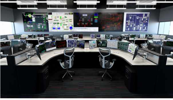
Command and Control Rooms
